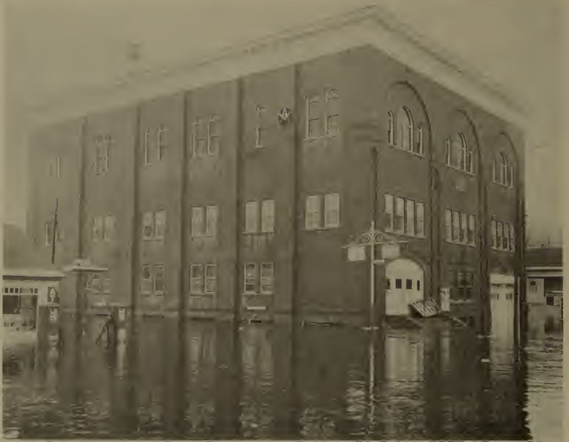
THE TOWN HALL BECOMES AN ISLAND AS OVER EIGHT FEET OF WATER ENTERS THE BASEMENT
