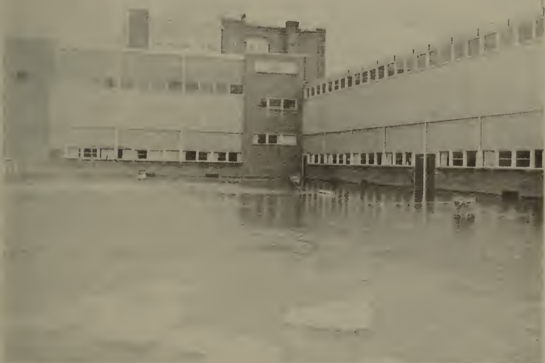
NO SCHOOL DURING THE FLOOD AS WATER ENTERS THE FIRST FLOOR
