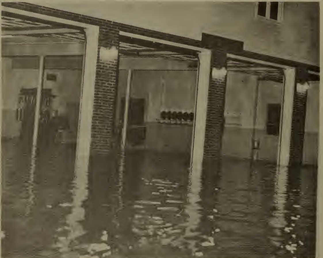
TWO FEET OF WATER COVERS THE COMPLETE FIRE STATION
