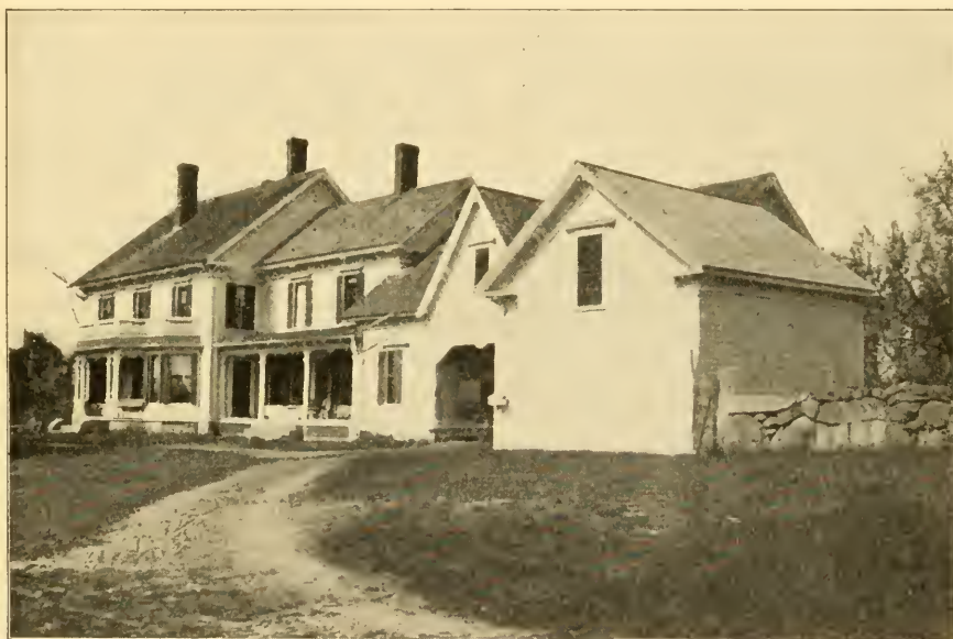
Residence of Charles H. Carpenter, Chichester
