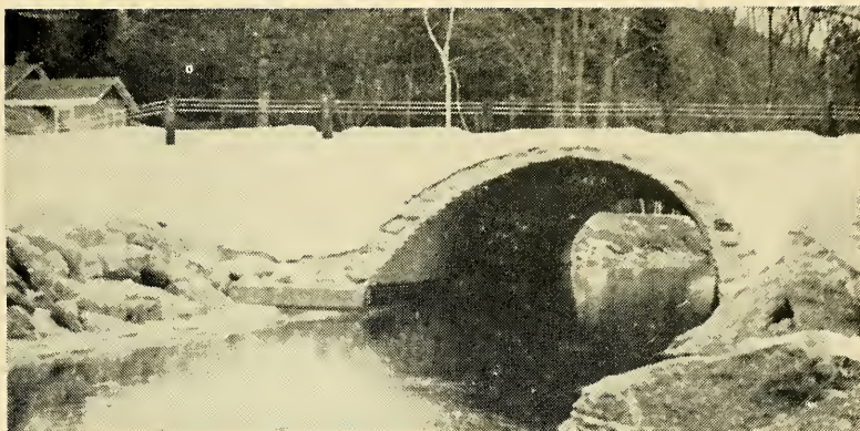
NEW BRIDGE AT REED'S OVERFLOW
