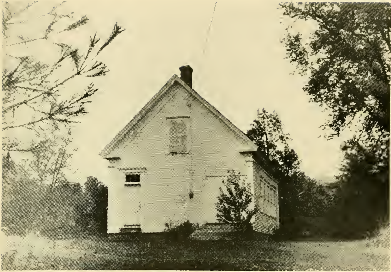
OLD CROYDON FLAT SCHOOL
