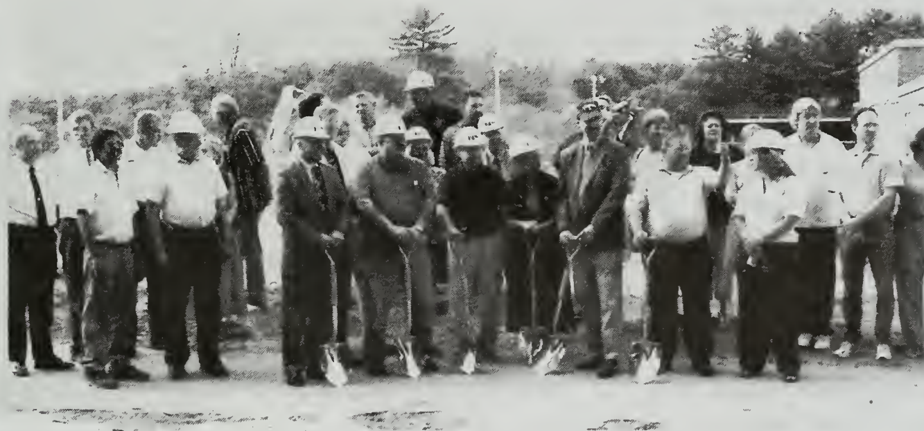
Groundbreaking Ceremony August 25, 2005
