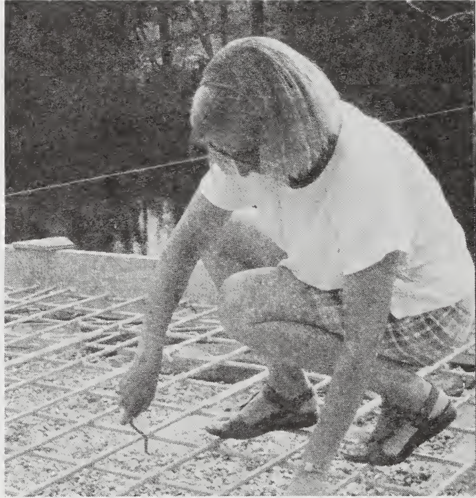
Margot Estabrook tying rebar Patrick O'Grady photo
