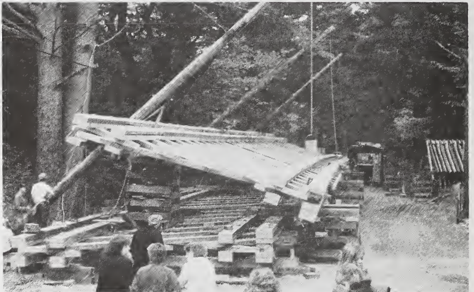
Raising the walls Andy Andrews photo
