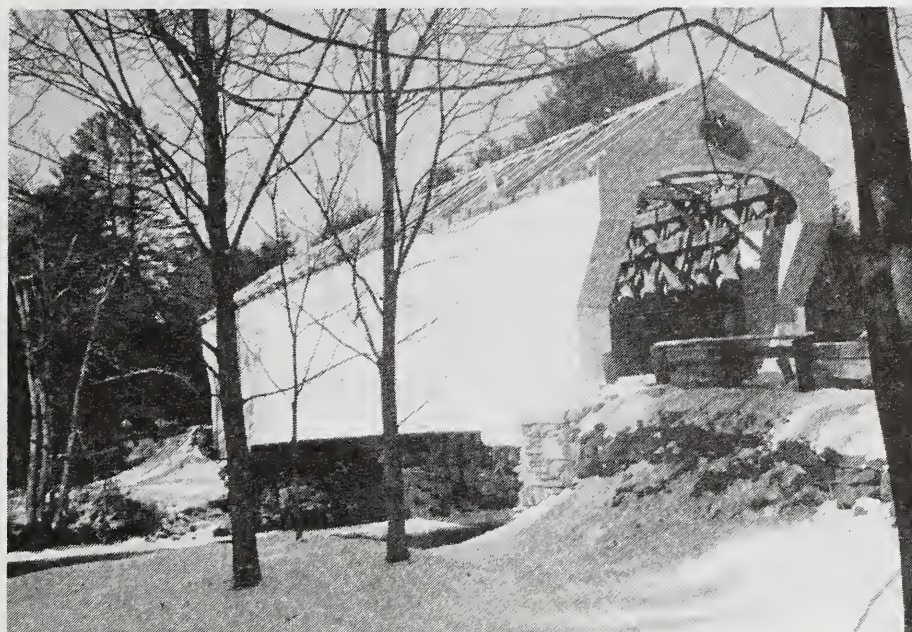
Winter has come and the bridge is almost done. Patrick O'Grady photo
