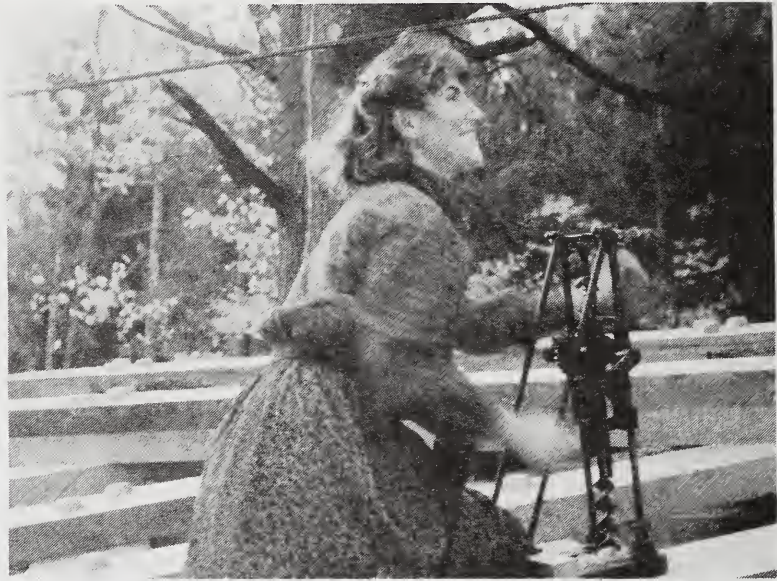
Gerrie Black, one of Newport's first citizens to step forward as an advocate, drilling holes for the trunnels. — Andy Andrews Photo
