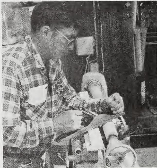
Arnold Graton fine-tuning one of 1200 trunnels used to hold the new bridge together. — Patrick O'Grady photo
