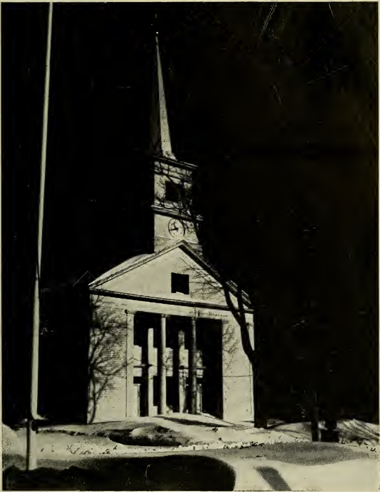
View of Community Church Showing New Clock War Memorial
