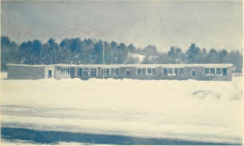
New Barnstead Elementary School
