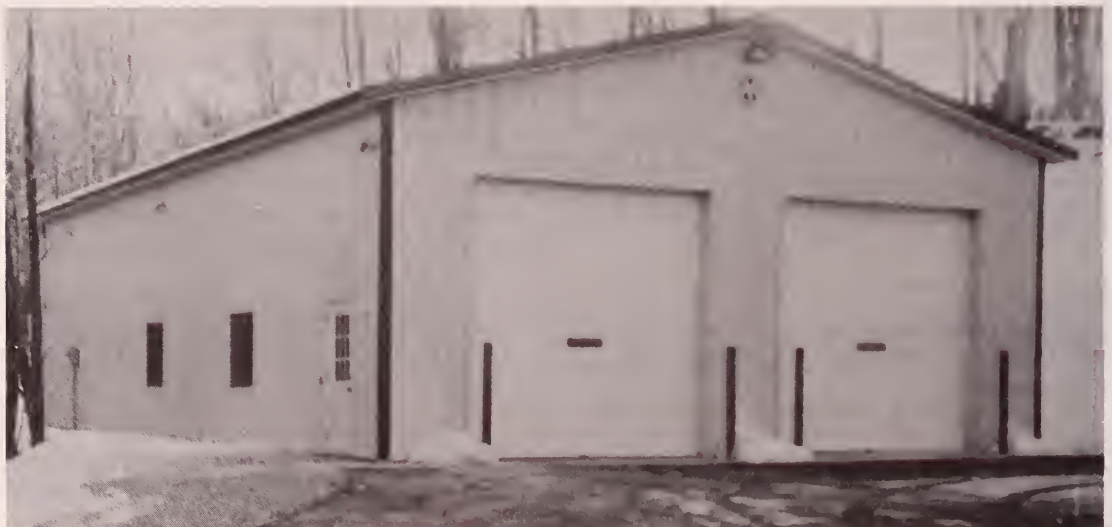
SOUTH WEARE FIRE STATION ROUTE 114
