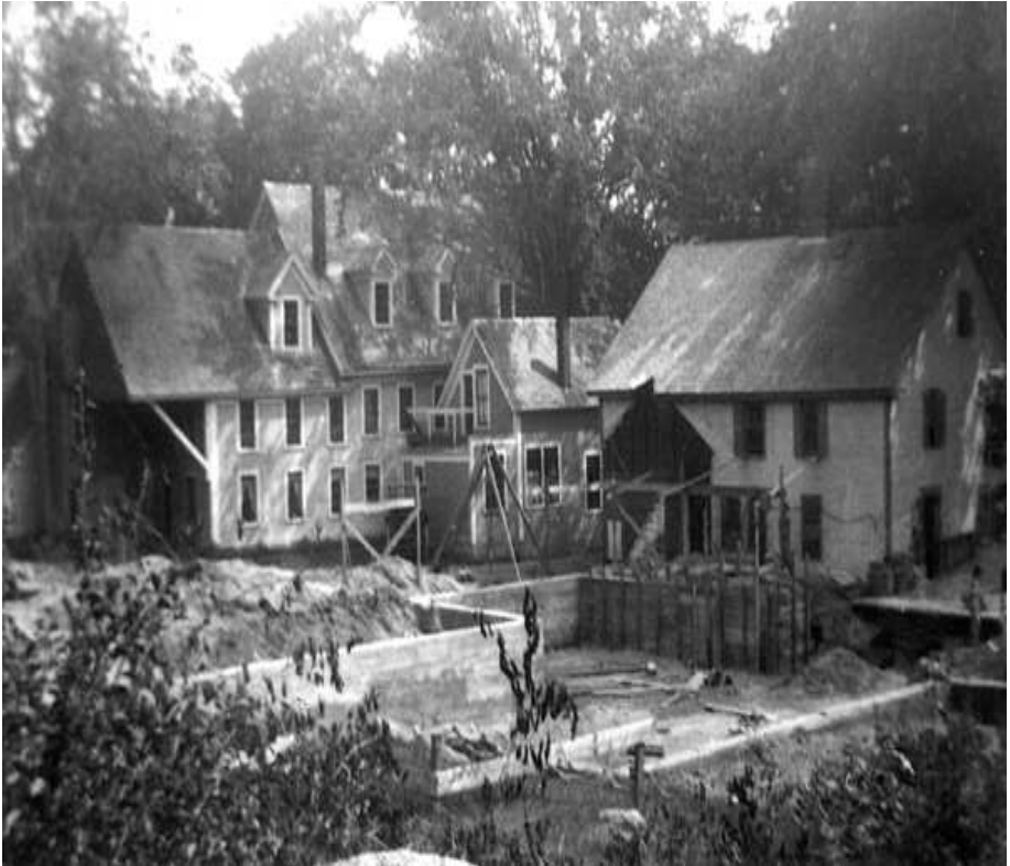
Construction begins for the new Town Hall.
