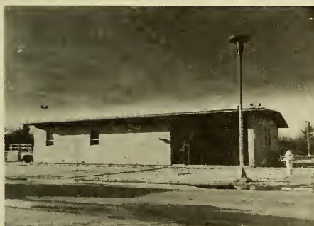
Sewer Treatment Plant
