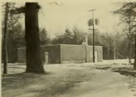
Pumping Station - Canobie Lake
