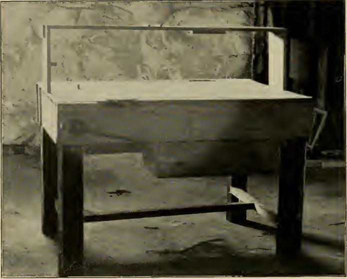
DOUBLE BENCH MADE TO ACCOMMODATE TWO PUPILS. Total cost, including two home-made vises, $1.75.
