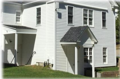
Library Lower Level Renovation 2014
