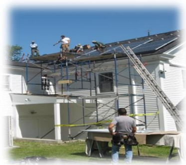
Solar Panel Installation 2015
