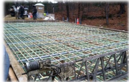
Bailey Brook Bridge Repair 2015
