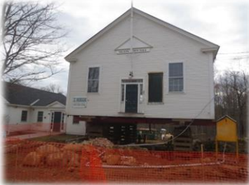
Town Hall Renovation 2014
