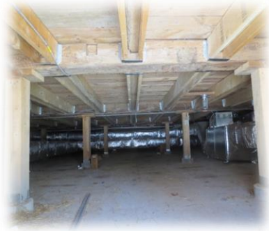
Town Hall Structurally Sound 2014
