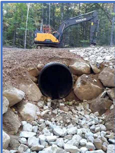
BURGDORF RD. STORMWATER CULVERT
