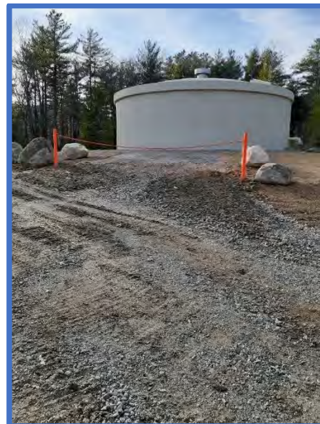
REINACH 120,000 GALLON TANK
