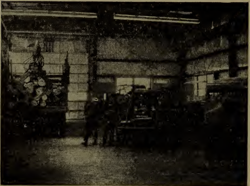
View inside shop looking to rear of building.
