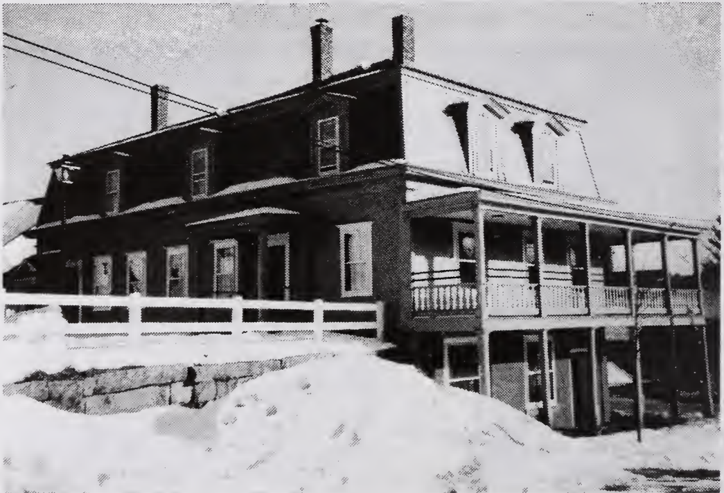
Kimball House built after the Cheshire Railroad came to Troy and served as a hotel for visitors. Today it is part of the Troy Senior Housing Complex completed in 1999.
