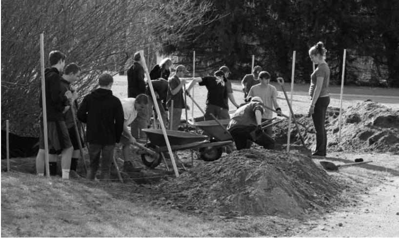
Mrs. Hemingway's KRHS Class preparing a "rain garden" to reduce the high school parking lot run off.
