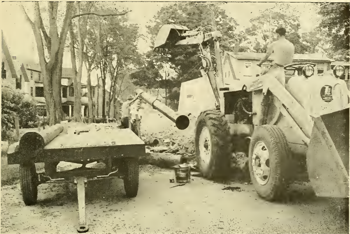
Water Department Laying 8" Main on Union Street
