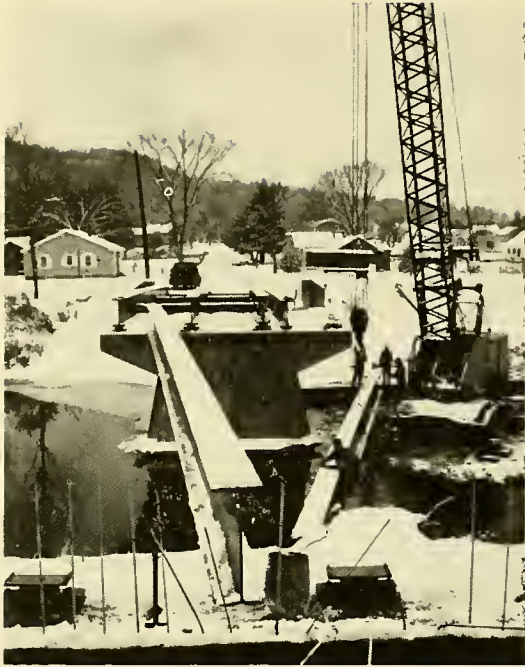
Beauregard Bridge Across Sugar River Under Construction
