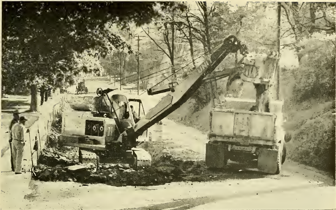
Highway Department Excavating Road Bed On Pleasant Street Reconstruction Project
