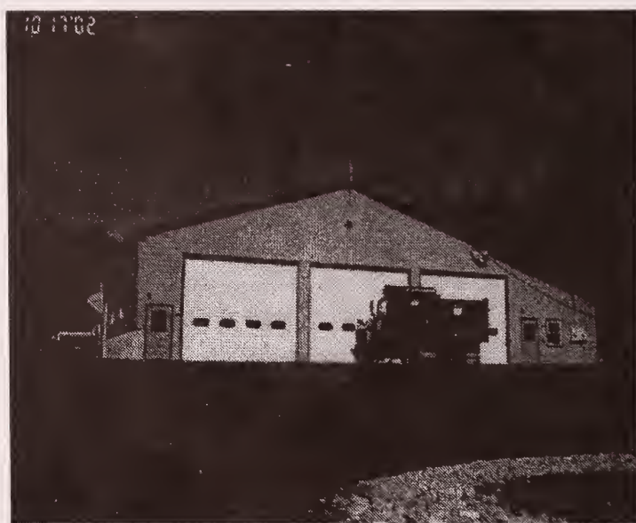
October 17, 2002 New Highway Garage Finished
