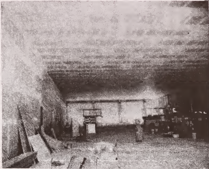
September 18, 2002 – Interior of Building Sheetrock and double ceiling going up
