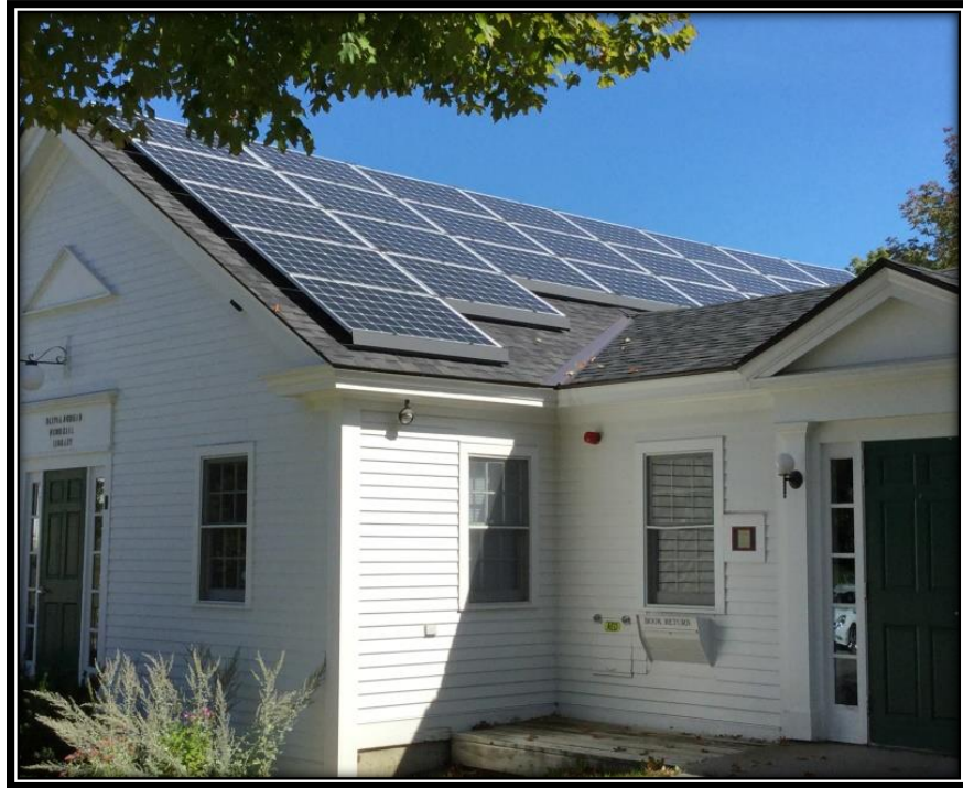
Solar Panels on Library Roof
