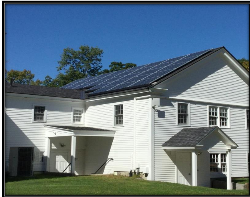
Rear view of Solar Panels on Library Roof
