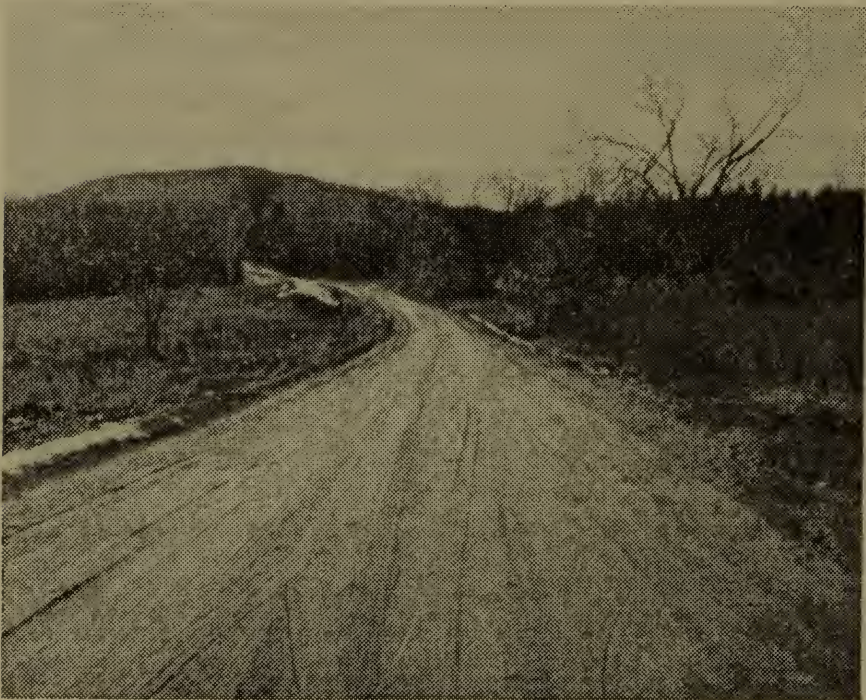
After reconstruction (near completion)
