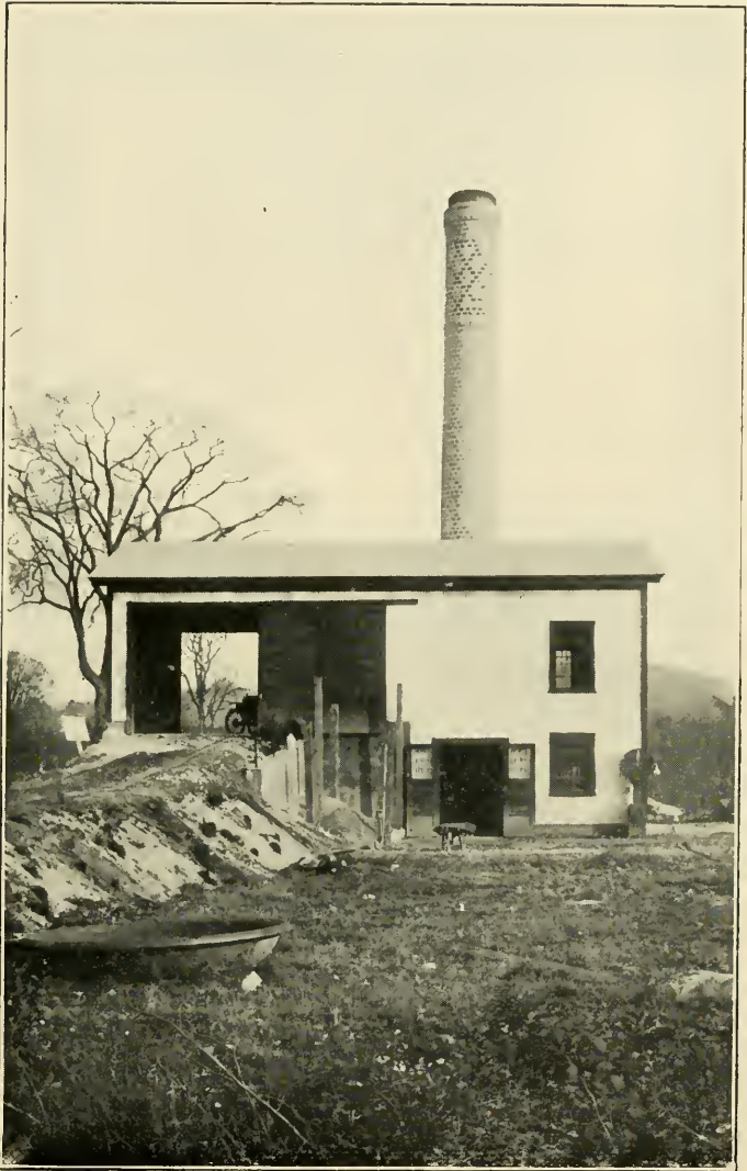
INCINERATING PLANT AND GARBAGE DESTROYER
