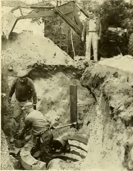
Highway Dpartment Constructing Drainage System.
