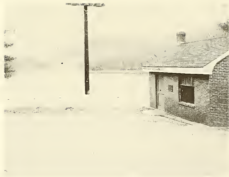
HOOKSETT VILLAGE Water Precincts pumping station and view of Pinnacle Pond.
