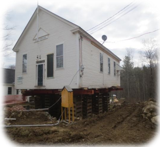
Front view of Town Hall fully raised to receive new foundation
