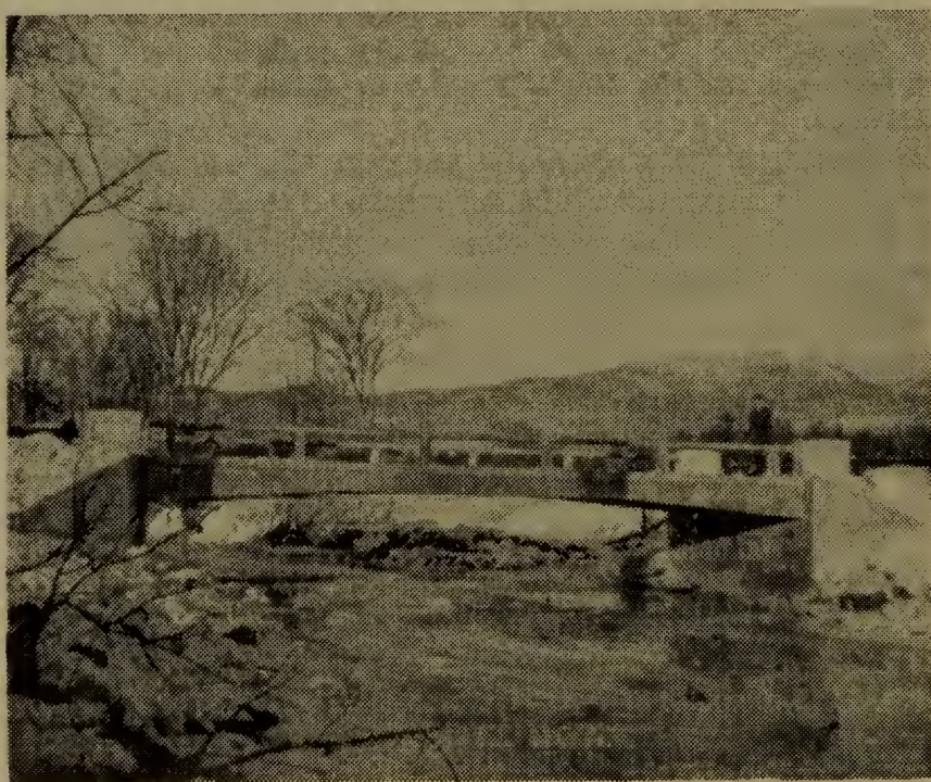
New bridge completed in November under State Aid Bridge Construction program.
