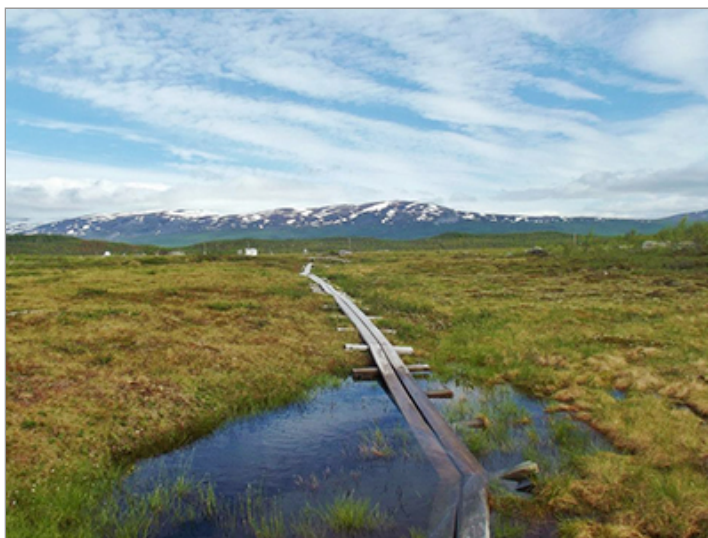
The boardwalk through the Stordalen Mire Nature Preserve in Abisko, Sweden. Part of it has sunken into a thaw pond due to thawing permafrost. Photo by Jessica DelGreco, UNH-EOS.
