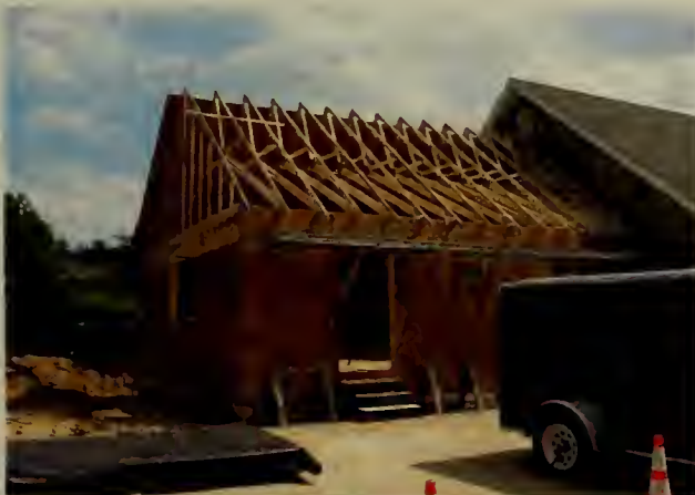
Library addition in progress, June 2007.
