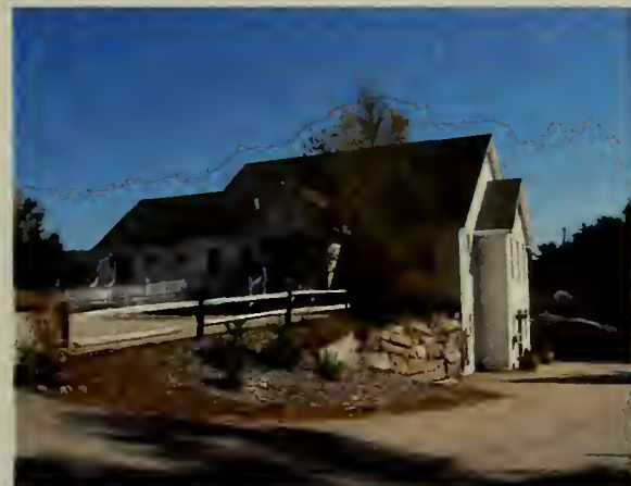
Rearview of Library with completed addition.
