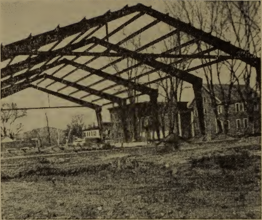
The frame goes up for the new town garage
