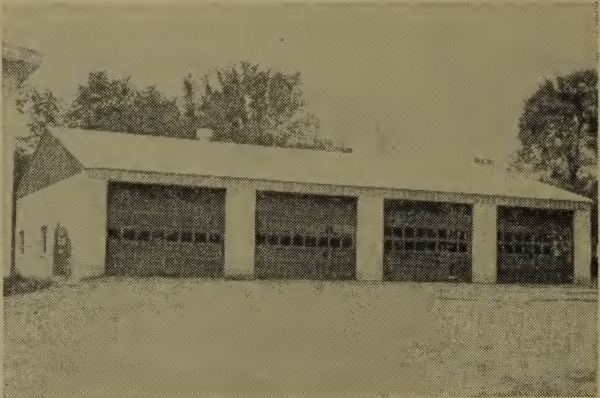
Completed, the garage houses 8 vehicles and other equipment
