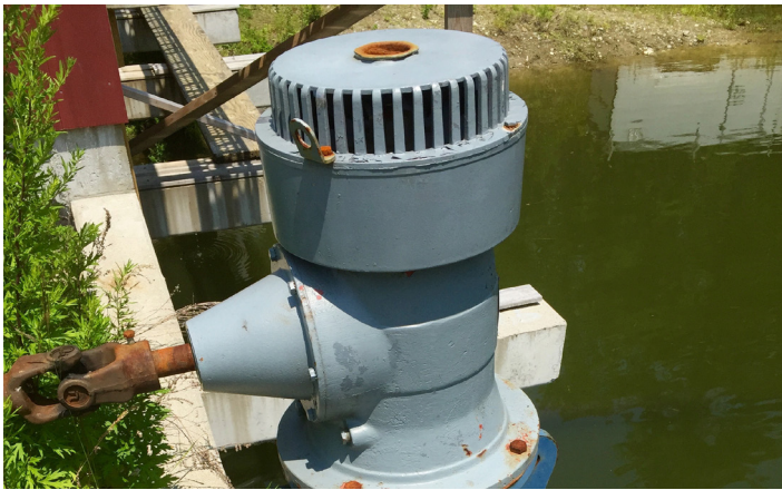
FIGURE 4: Water is the single most important resource in cranberry production. Through a USDA grant, the farm constructed a lift pump, reducing their cost to flood the bog from $400 to $50.
