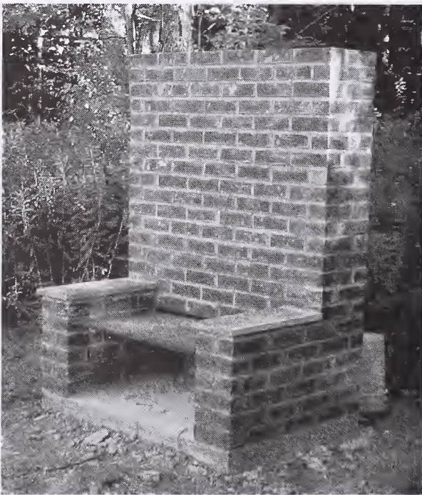
Outdoor fireplace constructed at the Hewes Field by resident Dan Rondeau as part of an Eagle Scout project. —R. Wheeler photo
