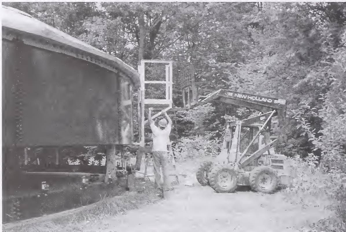
Workers installing the replacement tank for the Meriden Water District. The tank is built top to bottom with each new section built under the previous one.
