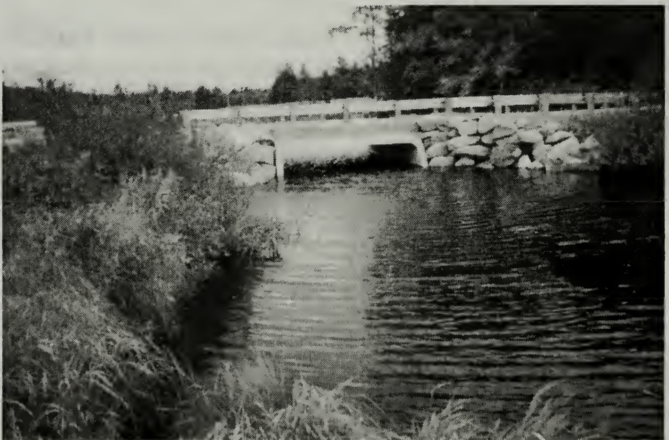
Penacock Road Bridge
