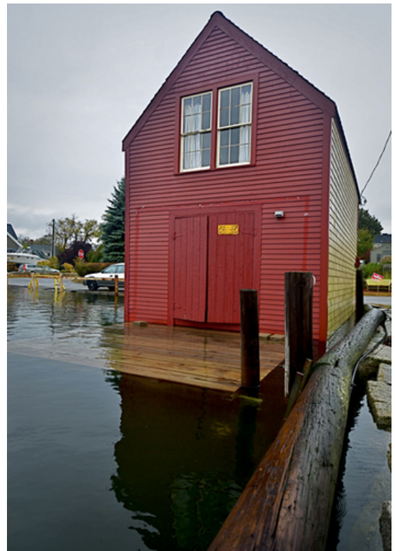
Today, infrastructure must be designed with "the explicit recognition that the climate is changing." Photo by Tim Hayes courtesy of Piscataqua Region Estuaries Partnership.
