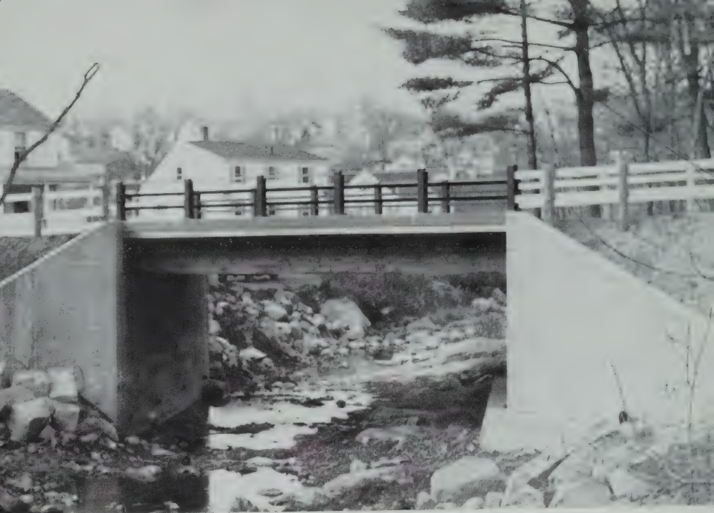
New Bridge — Spring Street to Glenwood Cemetery
