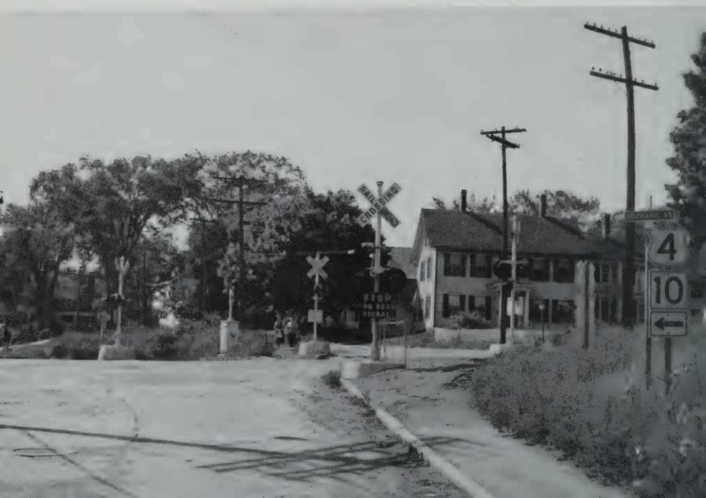
Looking West Mascoma Street Before New Construction
