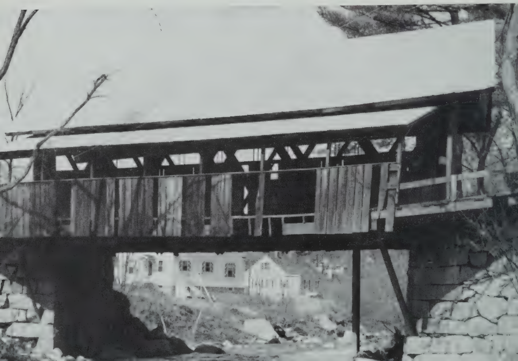
Old Bridge — Spring Street to Glenwood Cemetery
