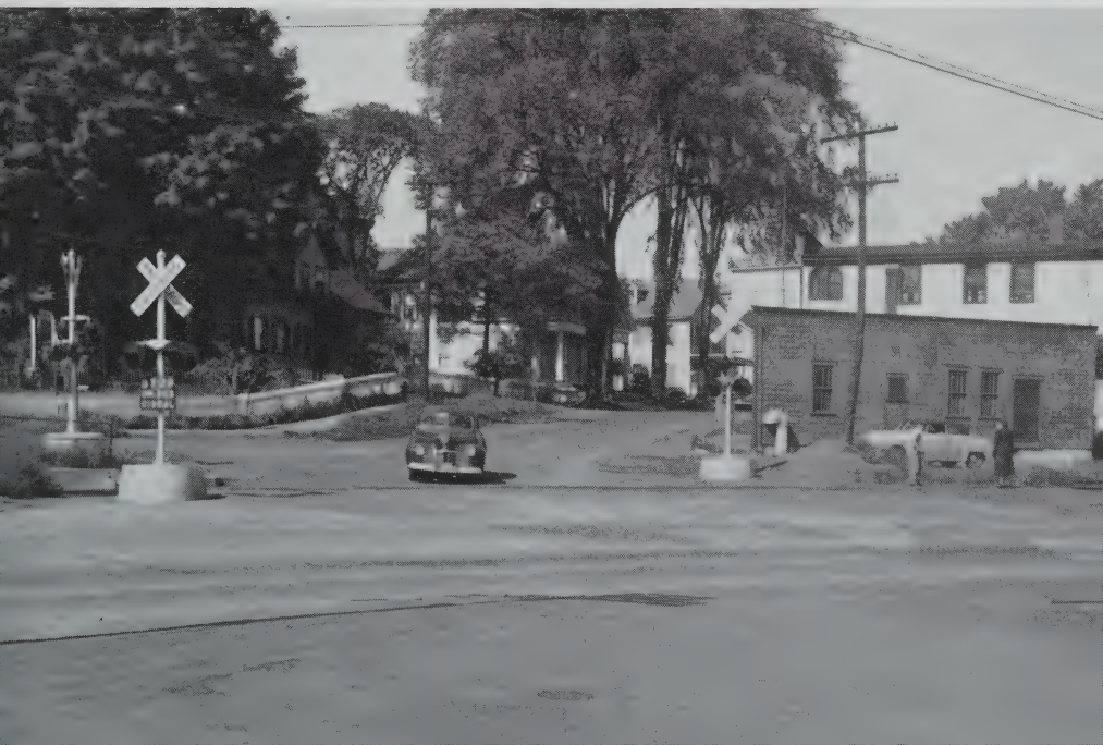
Jones Crossing Before New Construction
