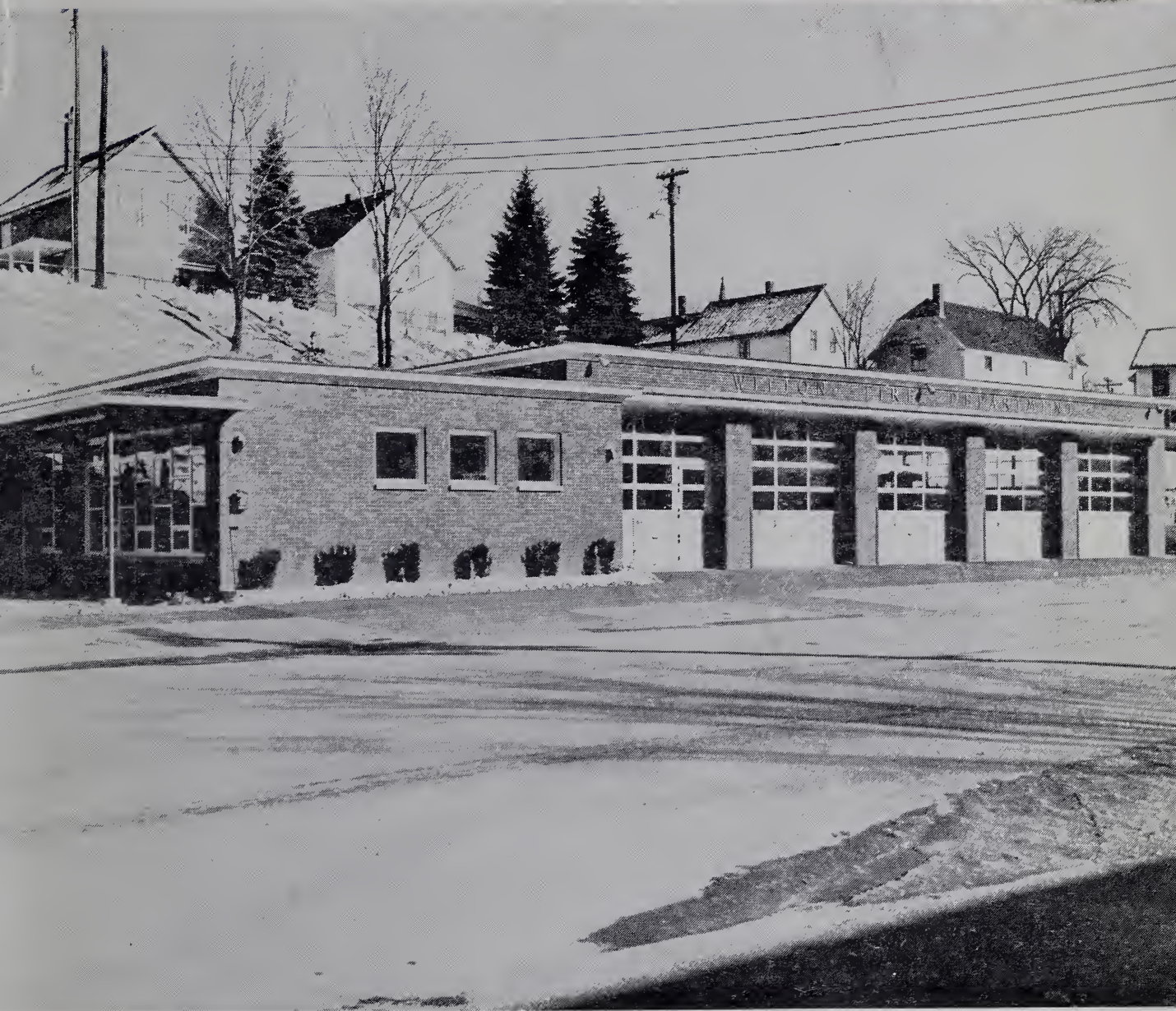
WILTON FIRE STATION
