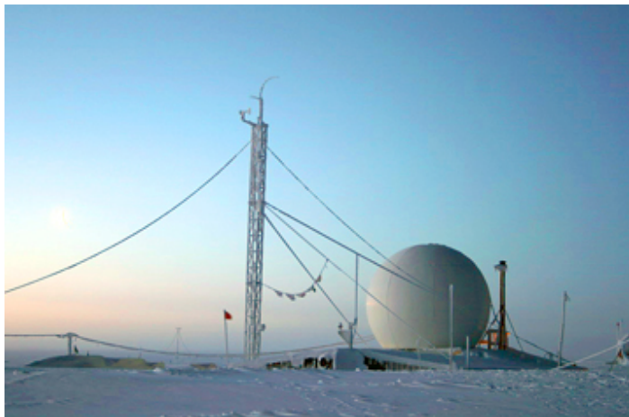
The main building or "Big House" at Summit Station. The dome houses the antenna for the satellite link to the outside world. Photo courtesy of John Burkhart, The Norwegian Institute for Air Research, Kjeller, Norway
