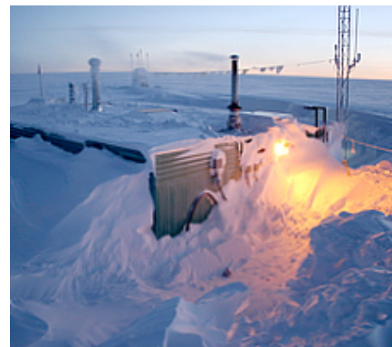
The Summit "berthing module" or sleeping quarters, which is the equivalent of three, combined office trailers with thickened walls to withstand the polar environment. Photo courtesy of John Burkhart.
