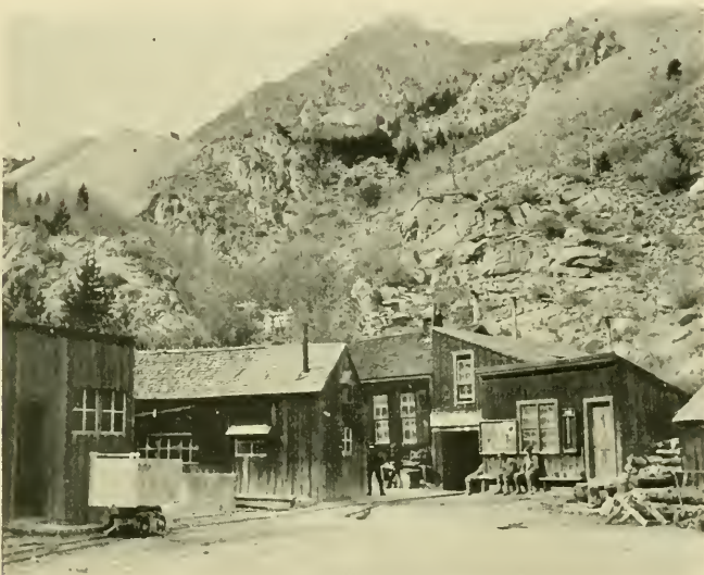
Entrance to Diamond Tunnel Mine, Silver Plume, Colorado.
