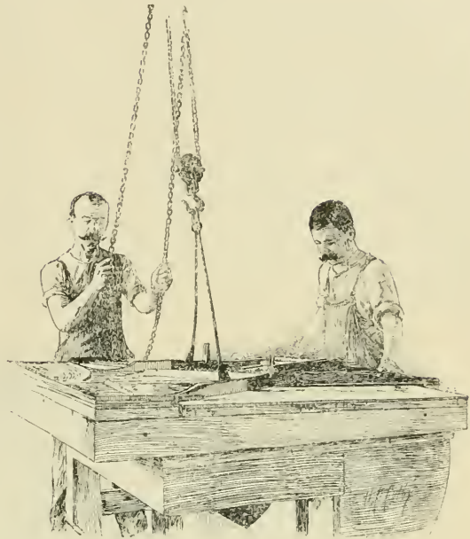
Placing Plate on the Form.
