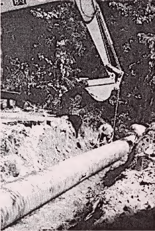
Highway crew laying culvert on Newbury Road.
