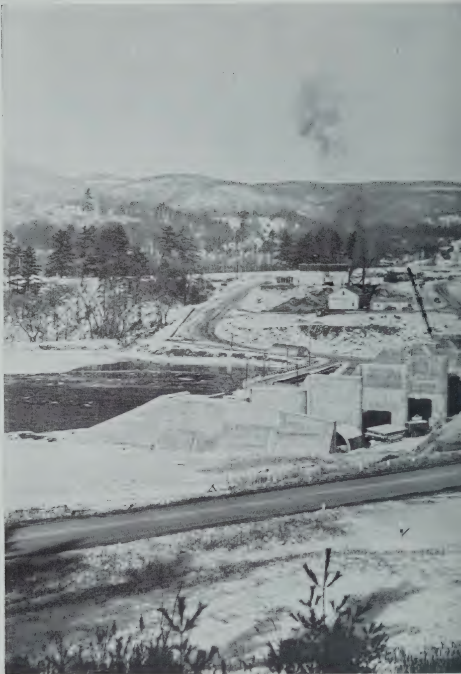
General view of Wilder Dam from the New Hampshire side. for completion in October, 1950. The 33,000-kilowatt plant will be owned by the Vermont Electric Power Corporation, Central Vermont Public Service Company, and will be connected to the power line to Bellows Falls. The insert at bottom, right shows the power plant under construction in January, 1950.
