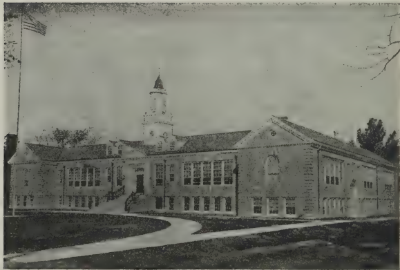
The Carpenter School
