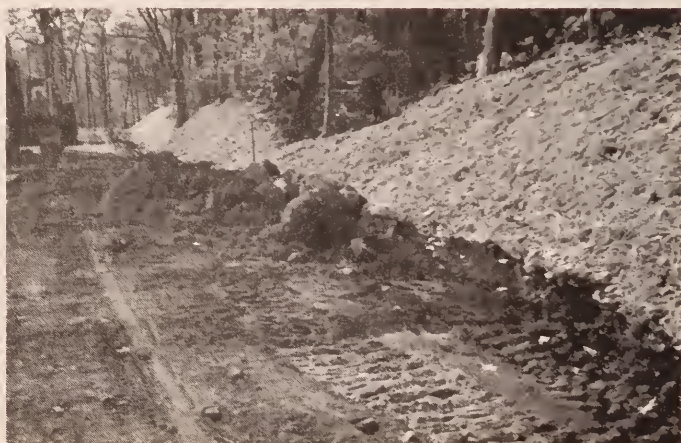
Embankment mulching after widening, Chalk Pond Road. (Capital Improvement Bond)
