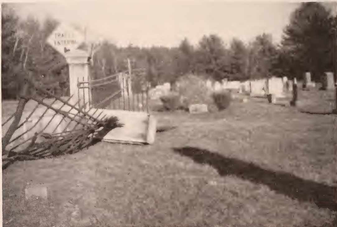
Damaged fence and granite posts, Millswood Cemetery. Restored 1990.
