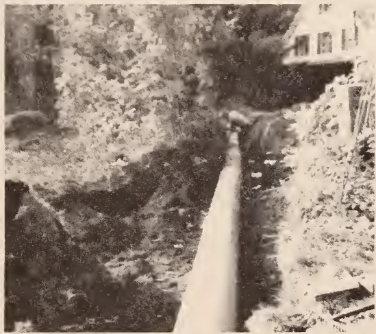
Keyser Street Improvement: (clockwise from above) Aticco machine behind grader, breaking up old pavement; aticco machine at work; the "pulverizer" makes large chunks into small ones; installation of culvert running from catch basin to Keyser Lake, at Gebbert property.
