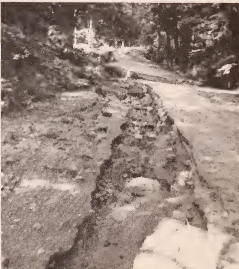
Culvert being installed on the Barker Road, replacing a wooden bridge.
