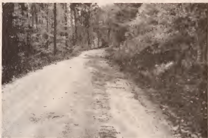
Widening, Chalk Pond Road, preparatory work. (Bond)
