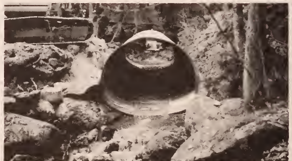
Culvert being installed on the Barker Road, replacing a wooden bridge.
