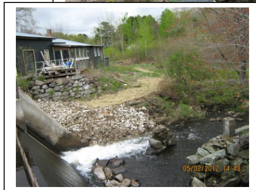
Downings Dam Work
