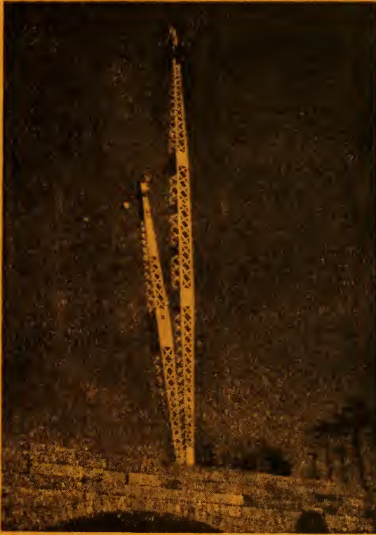
GUY DERRICK USED IN REBUILDING EDNA DEAN PROCTOR MEMORIAL BRIDGE
