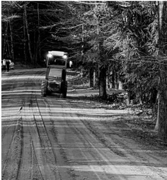
Above: New roller compacting Whitney Brook Road.
