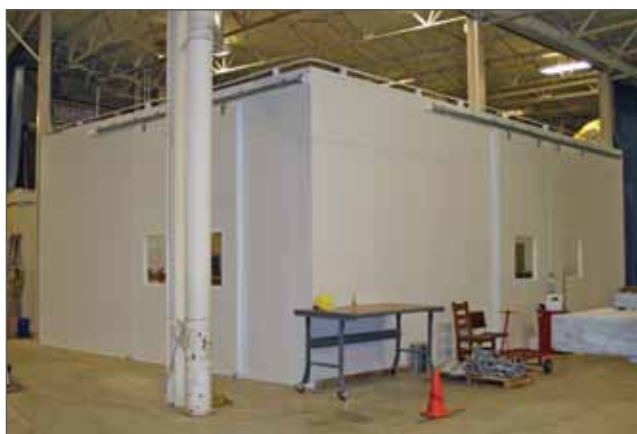
Figure 1-12. New room constructed in the high bay for ROV storage.
