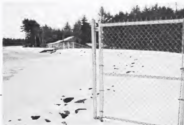
March's Pond Dam
