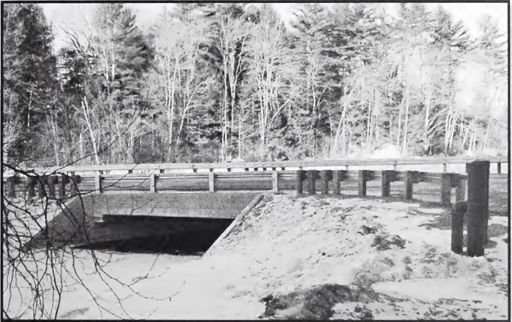
Davis Crossing Road new culvert installed December 2009
