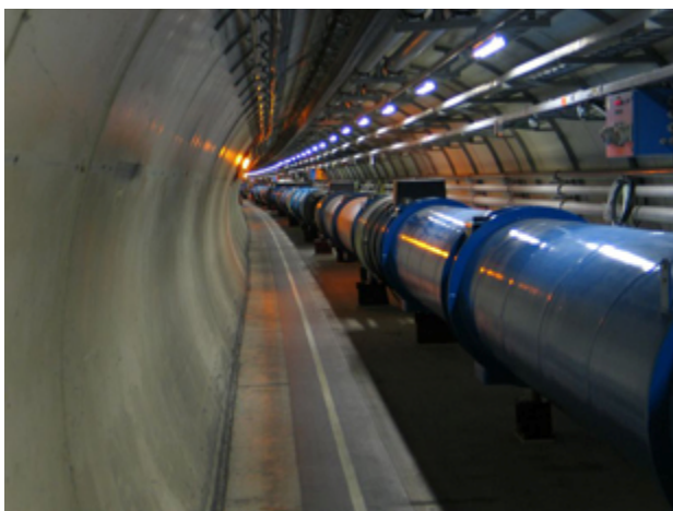
Figure 2. The LHC tunnel is large enough for a person to stand up inside. Two hadron beams will circulate in opposite directions inside the blue tube in the center of the tunnel. Image courtesy of LHC Machine Outreach, http://lhc-machine-outreach.web.cern.ch .
