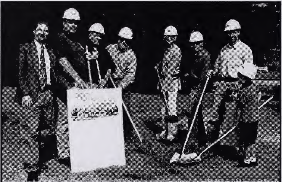
Peter Tennant, architect; John Bruss, Bruss Construction; Richard Wright, James Powell, Barbara Freeman, Del Harris, and Gary Budd with his helpers break ground for the new addition to the Town Office on August 7, 2004. Photo courtesy Shelly Candidus
