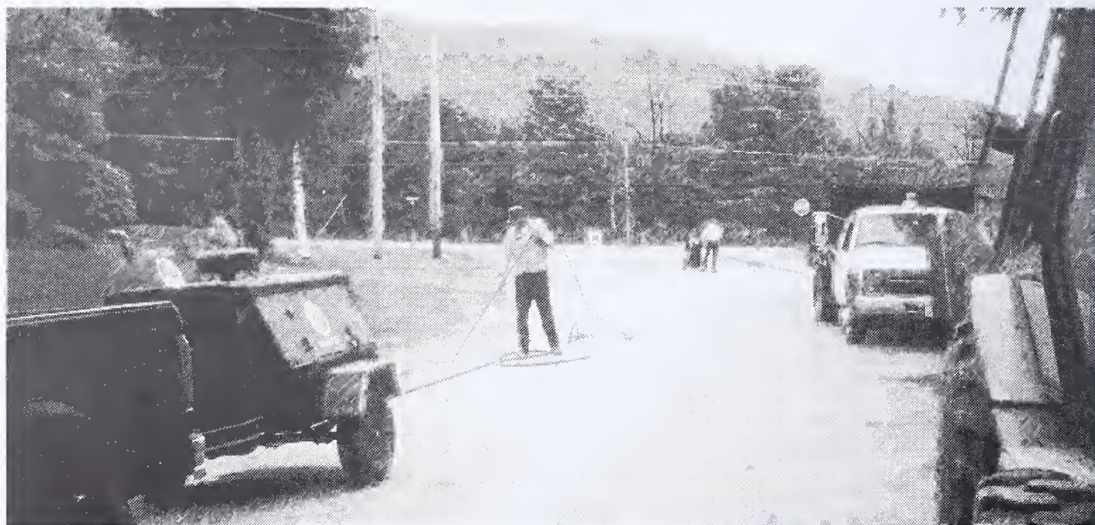
Crack Sealing By Public Works Department
