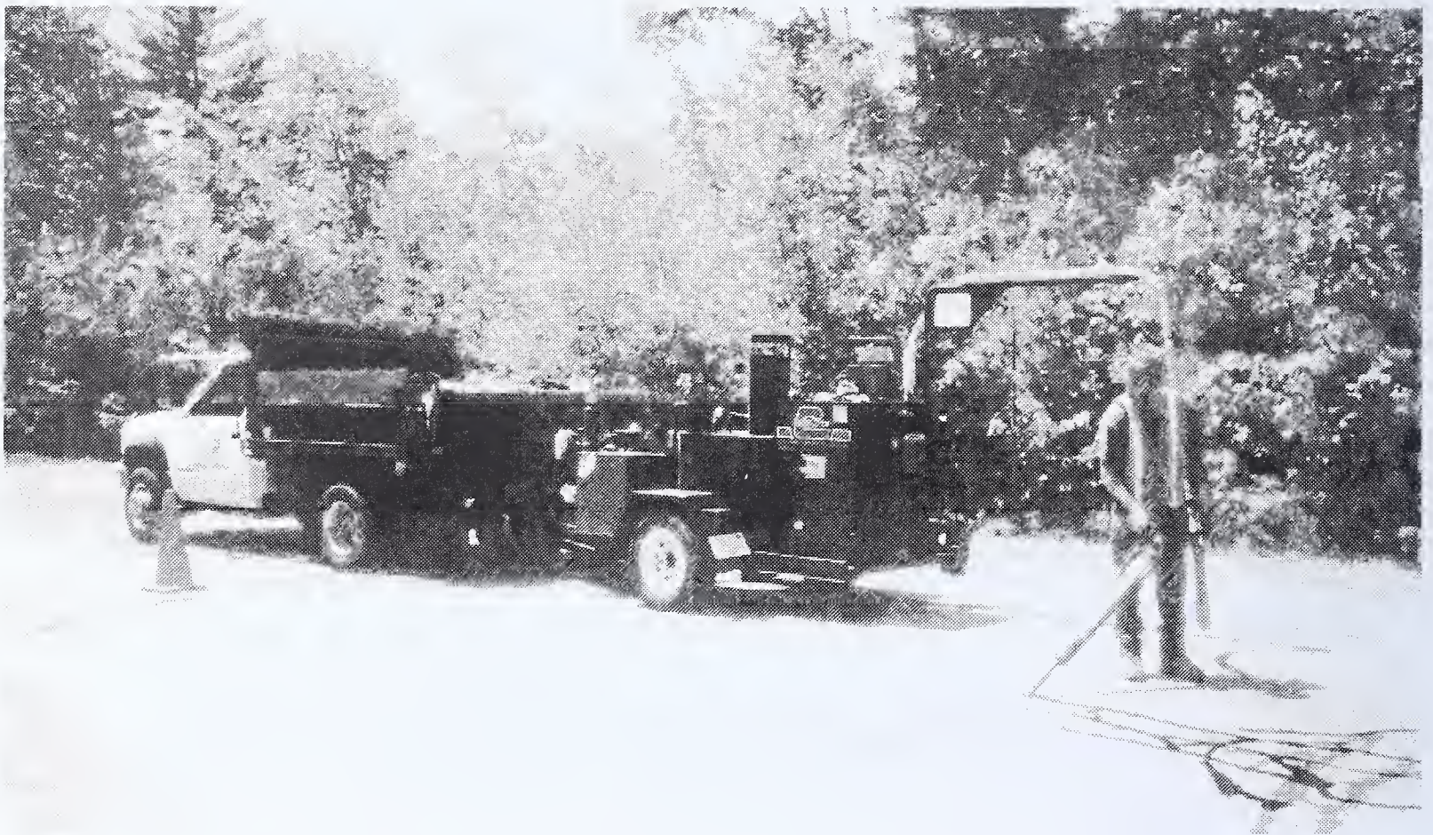
Department of Public Works Repairing Cracked Asphalt
