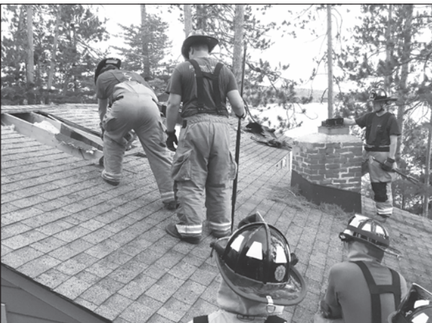
NLFD Firefighters were lucky to train in a donated building. They are practicing how to properly vent a roof. Photo courtesy of NLFD.
