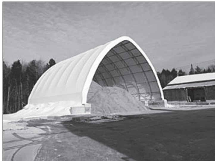
The new sand & salt shed at the Public Works Department.
