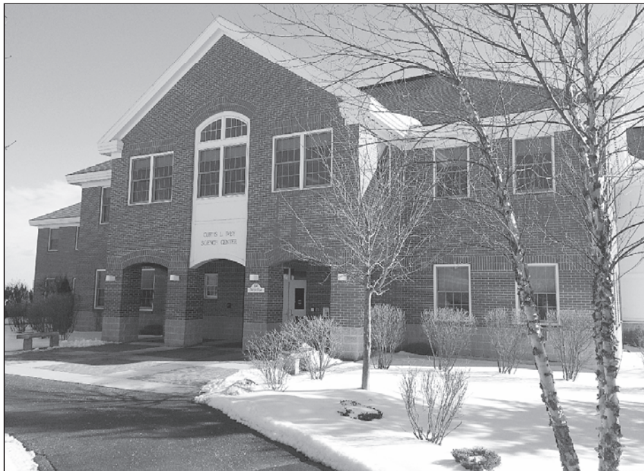
The Curtis L. Ivey Science Center is Colby-Sawyer's first new academic building in four decades. The 33,000-square-foot building houses the Community and Environmental Studies and Biology Programs, as well as faculty in the Natural Sciences Department.
